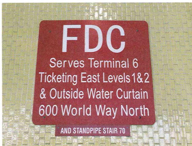
FIGURE 15-6 When standpipe FDCs serve more than one building or location, signage should be provided for the buildings and locations served.
