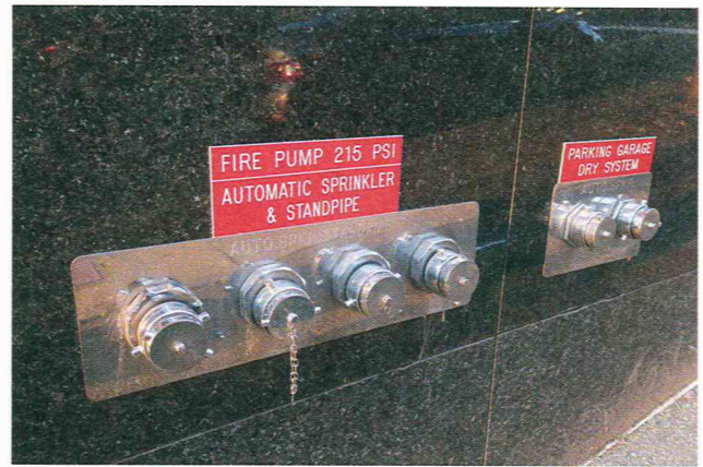
FIGURE 15-5 The fire code requires standpipe and sprinkler FDCs to be labeled. If there is signage for pressure requirements, pump to the posted pressure.
