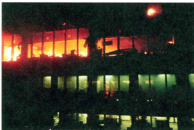
FIGURE 15-46 The fire conditions on floor 12 of the First Interstate building are clearly visible. Light smoke is visible on floor 11, with what appears to be a trapped occupant shrouded by smoke.
