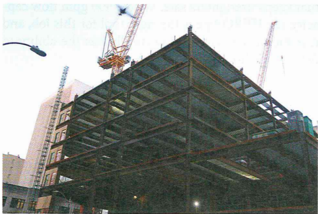
FIGURE 15-52 By exposing the steel I-beam grid above them, firefighters can place themselves in the right spot to use a concrete-cutting tool on the Q-decking from the floor above the fire, then drop distributor nozzles into the fire area.
