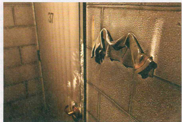
FIGURE 15-7 The floor 37 placard melted from the heat on floor 36 at the DeWitt-Chestnut Fire in Chicago, Illinois.
