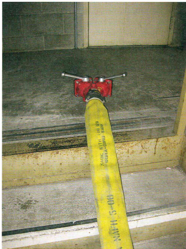
FIGURE 15-39 To limit the lengths of hose connected in the firefighting stairwell, a 2½-inch hose line can be connected to the standpipe outlet four floors below the fire. This creates a second standpipe in the firefighting stairway.
