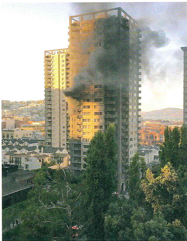
FIGURE 15-37 Although exterior windows failed in the Gateway Apartments and Townhomes Fire, the prevailing winds were light. A perfect scenario for a wind-driven fire was averted.
