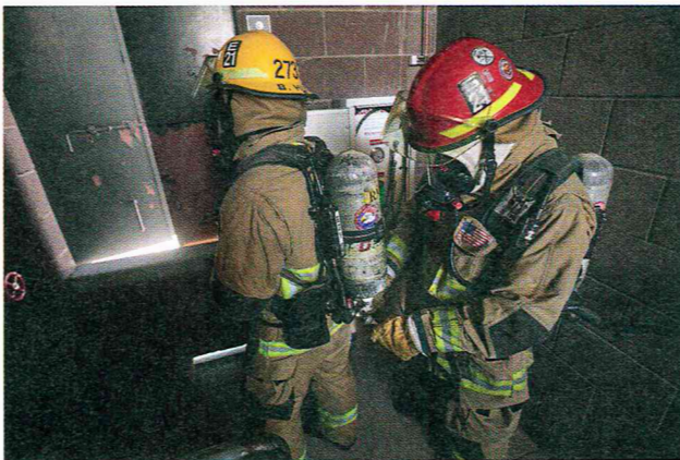
FIGURE 15-60 The firefighter air replenishment system (FARS), or the air standpipe, can be supplied by the building's cascade unit.
