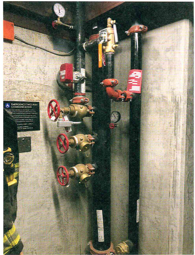
FIGURE 15-42 New standpipes have two separate 2½-inch discharge connections on each floor permanently affixed to the standpipe, thus creating a 2½-inch gated wye.
