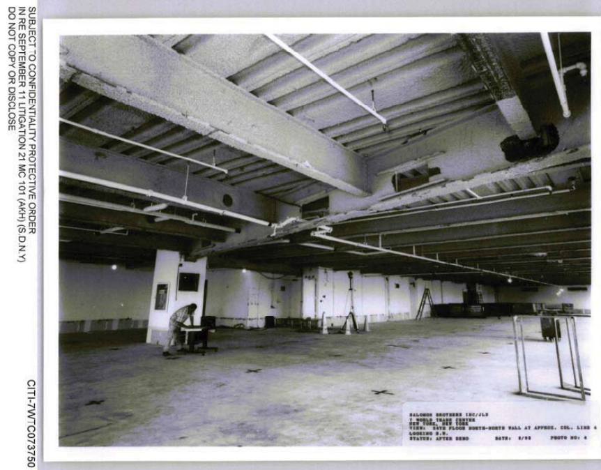
Figure A16 Photograph on 24 th floor showing unfilled flutes above girder
