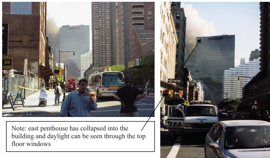
Figure 1 WTC7 before collapse (left) and during collapse (right)
