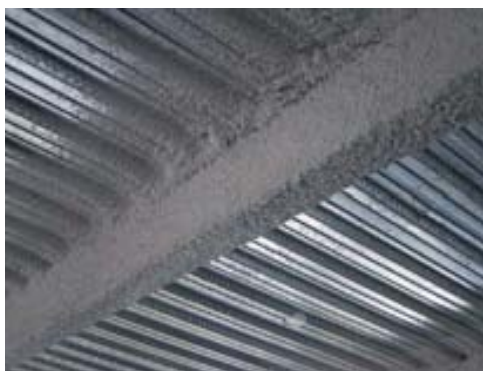
Figure C2 Voids filled with SFRM
