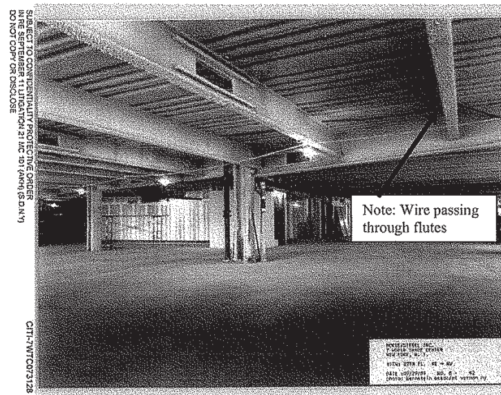
Figure A3: Photograph showing wire placed through flutes (29 th Floor).
