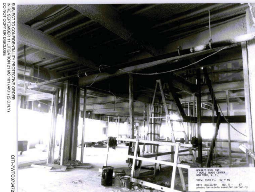
Figure A10: Photograph showing wire placed through flutes (35 nd Floor)
